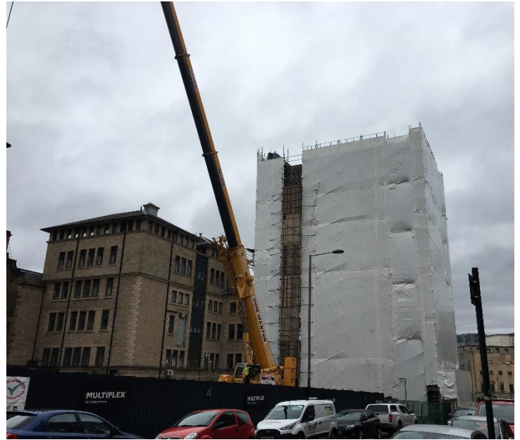
Structural demolition of the Pontecorvo Building
